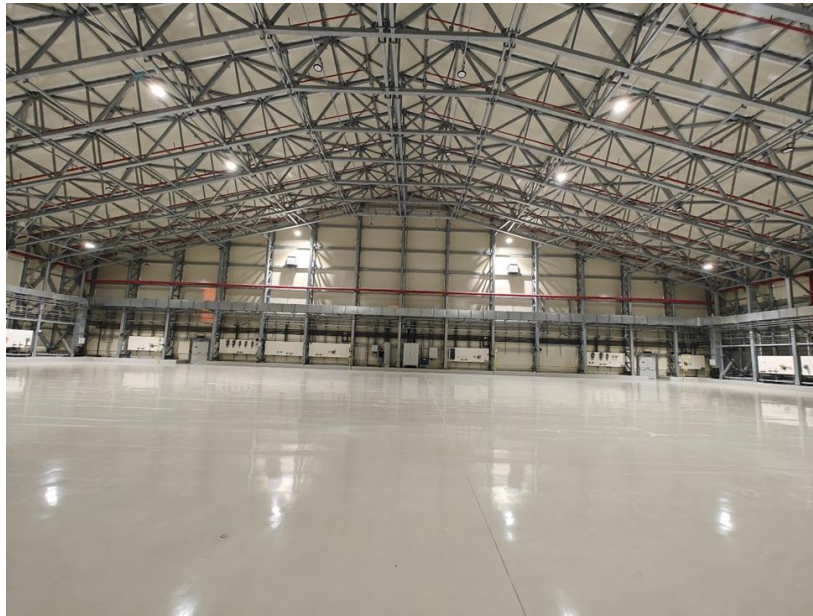
Figure 19. Maintenance hangar at the Athens International Airport
